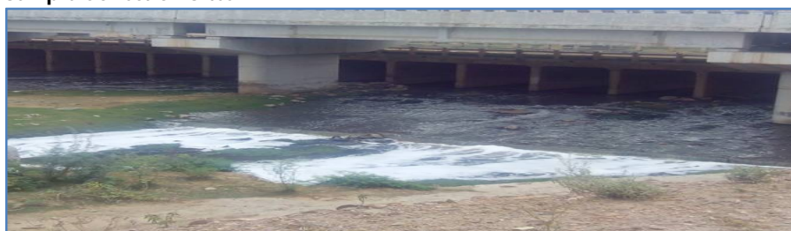
Fig 1(A)Sitapura Industrial area Site
